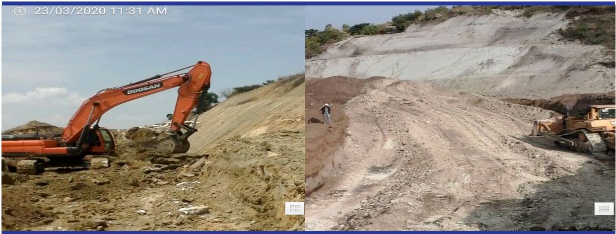
Partial Shikute-Chullute Asphalt Road Project Pictures
