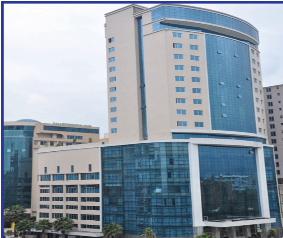
Completed Ellilly Multipurpose 24 Stories Building
