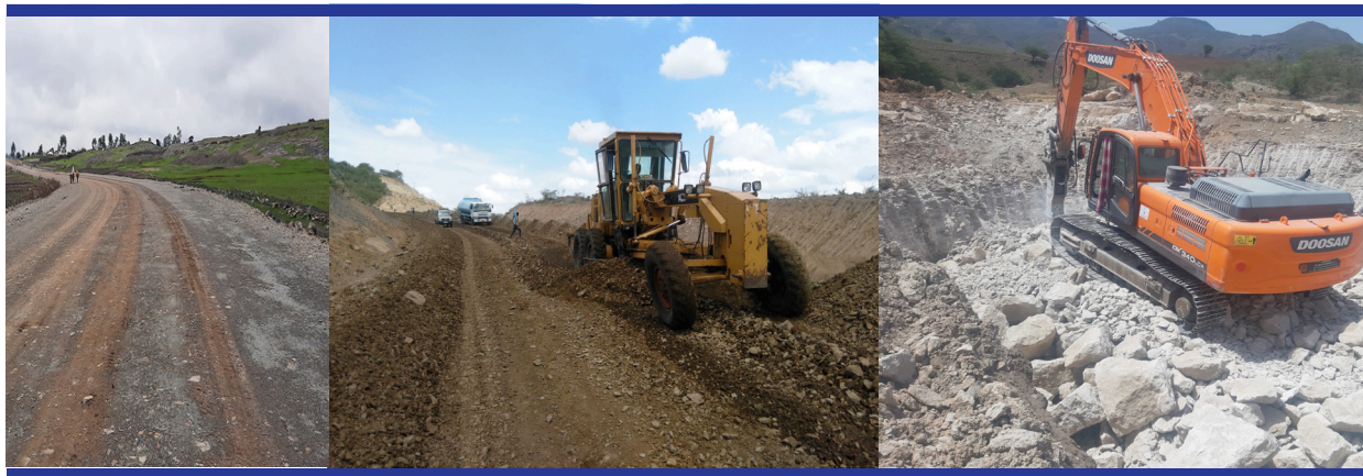
Prtila Picture of Alemketma -Degolo Asphalt Road Project at Different Stage
