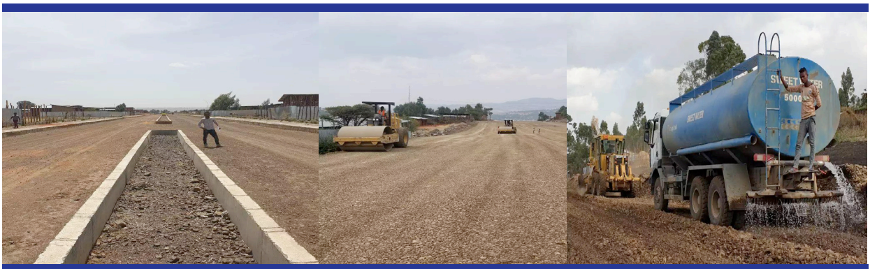
Ambo Town Internal Asphalt Road Partial Pictures
