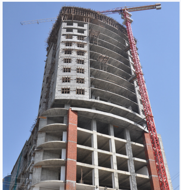
Elilly Multi-purpose Buliding Complex (Front View)
