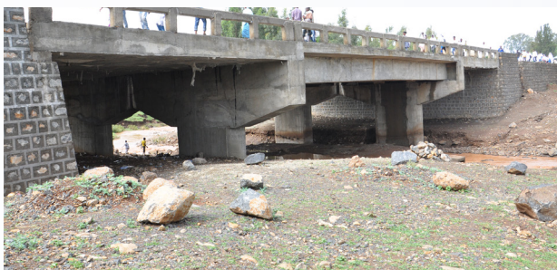
Completed 3 Span Girder Bridge
