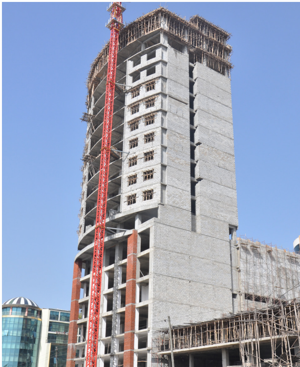
Elilly Multi-purpose Buliding Complex (Side View)
