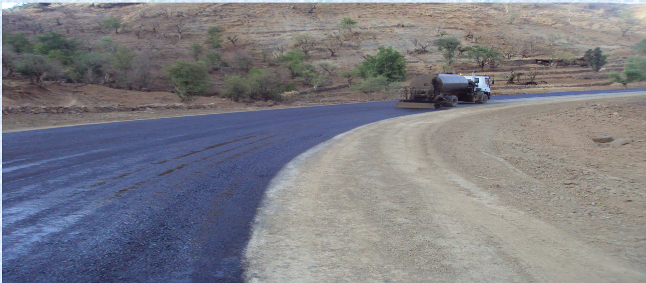
ማይፀምራ-ዲማ በግንባታ ላይ/Mytsebri -Dima While Under Construction
